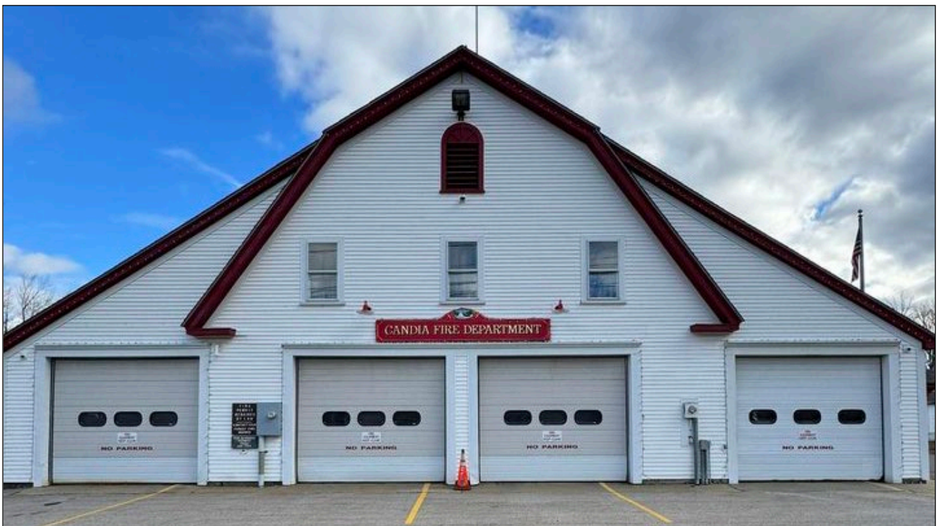
The Candia Fire Station has significant safety deficiencies, including no ventilation system for vehicle exhaust.
