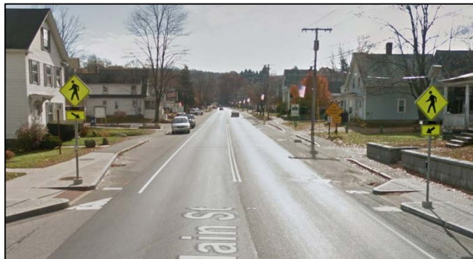
An Example of an Existing RRFB located in the Town of Marlborough, NH at a Mid-Block Crossing of NH Route 101
