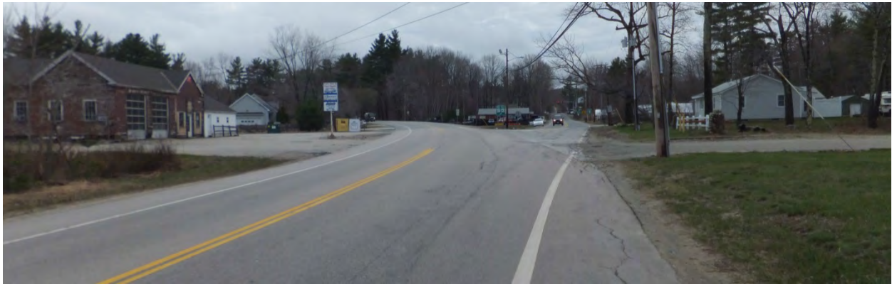
View of NH 27 looking west toward High Street. Photo shows two access points, one on either side of the road, that are located within the intersection.
