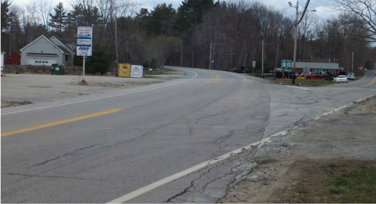
View of the intersection looking southwest toward Raymond Road (left) and High Street (right). Photo shows the wide expanse of pavement without markings within the intersection. Photo also shows the edgeline continuing from westbound NH 27 onto High Street.
