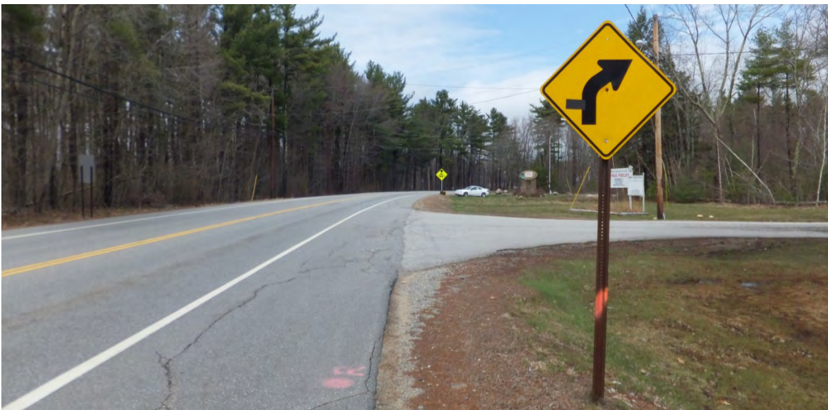
View of Raymond Road looking northeast toward High Street. Photo shows the existing intersection warning sign for High Street that is incorporated with the curve warning sign.
