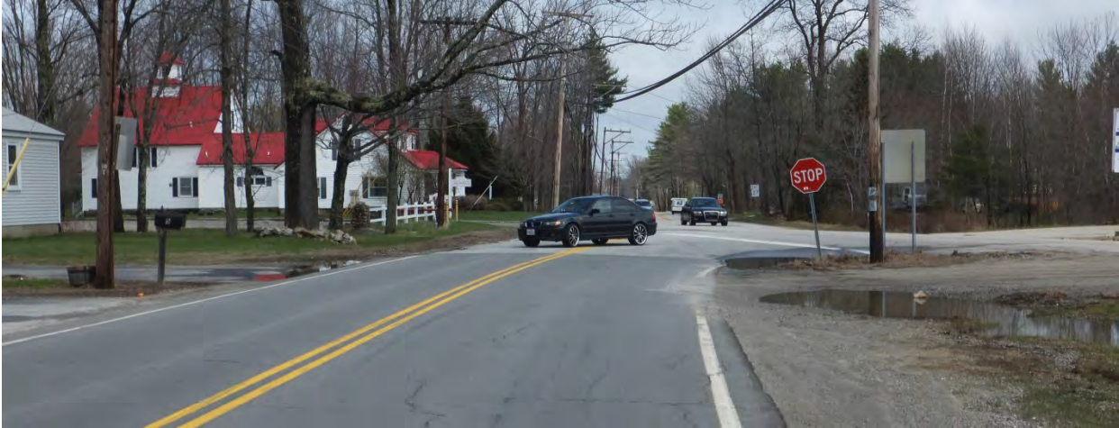
View from eastbound High Street approach looking east toward NH 27 and Raymond Road. The photo shows the severe skew of the intersection. Photo also shows a passenger car tracking into the opposing lane as it turns left from Raymond Road.
