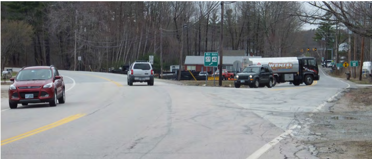
View of the High Street intersection looking west. Photo shows the skew of the intersection and limited sight distance to the southwest along Raymond Road due to the horizontal curve. The photo also shows a truck using an unofficial dirt path between High Street and Raymond Road to turn left from Raymond Road.
