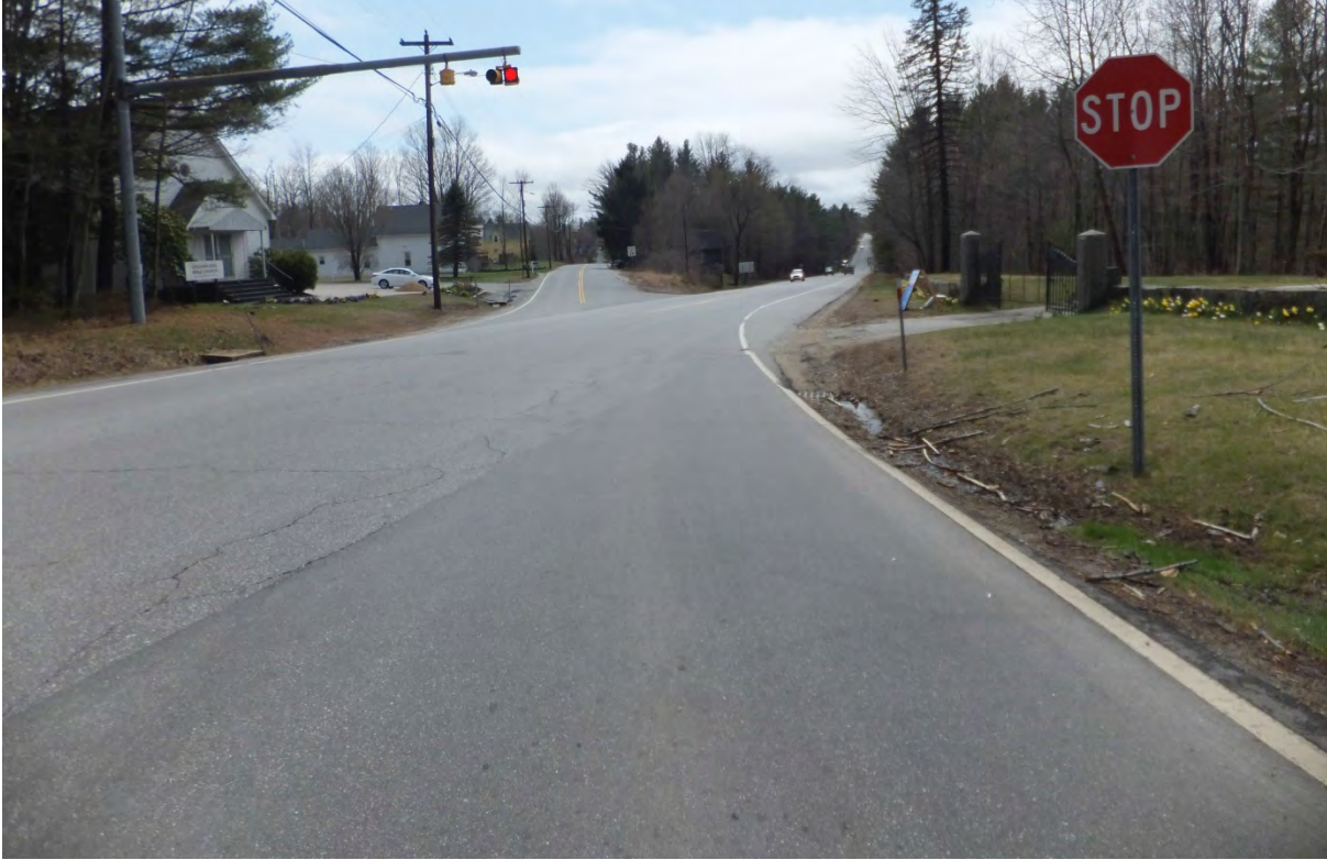
View of the intersection looking south from Main Street. Photo shows the extensive pavement within the intersection that is not defined by pavement markings.
