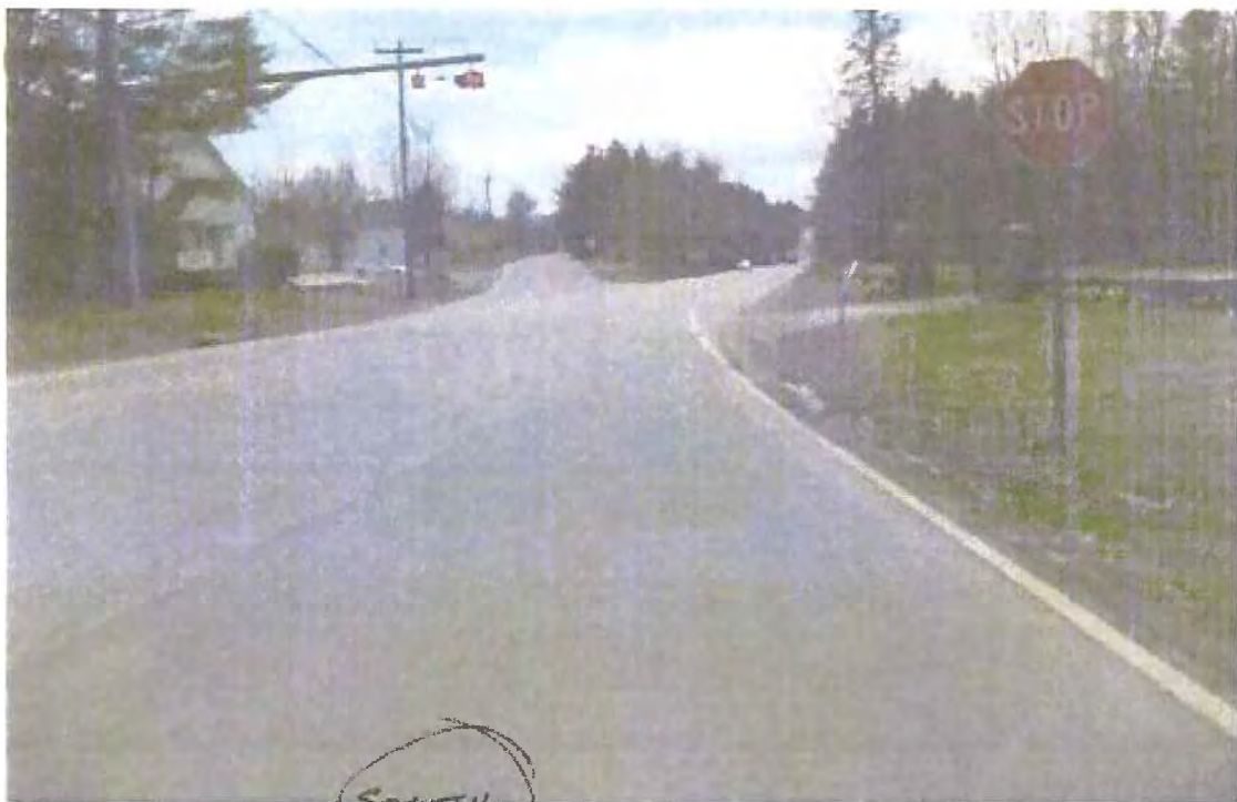
View of the intersection looking north from Main Street. Photo shows the extensive pavement within the intersection that is not defined by pavement markings.
